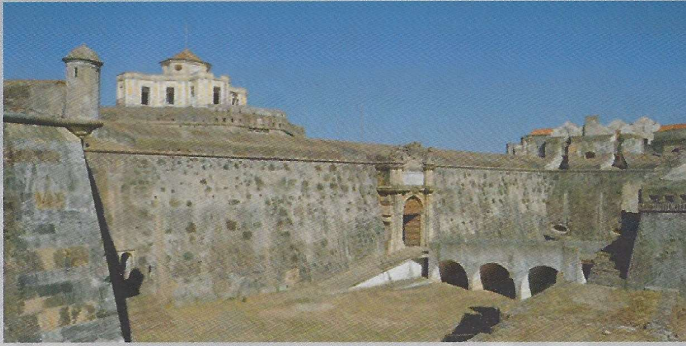
First ditch and the access to the inner gate
