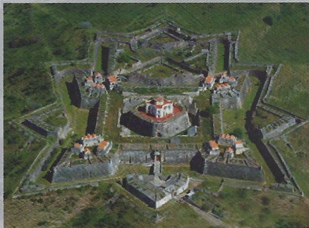
Aerial photograph (from S to N) (CME)
