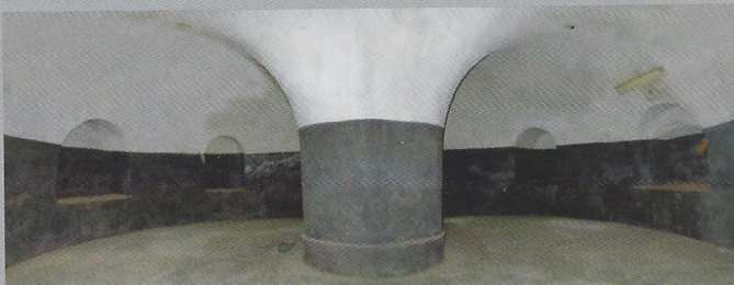
Guard-house in the passageway of the main gate
